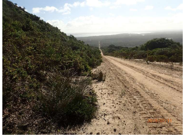
Figure 3: Photo of the vegetation within haulage road. The haulage road is the existing fire break and requires additional clearing (approximately 1 metre) along left hand side.
